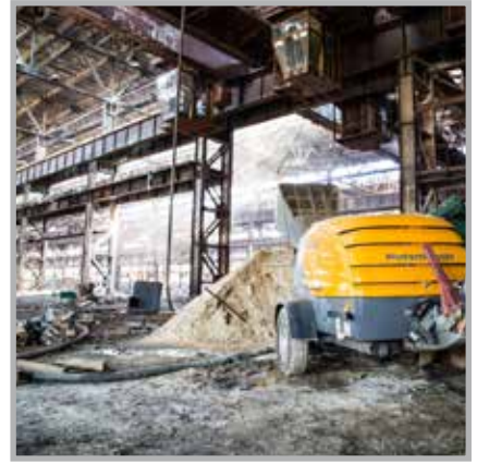
Russia, Ryazan placement of ~ 100,000 m 2 of screed
